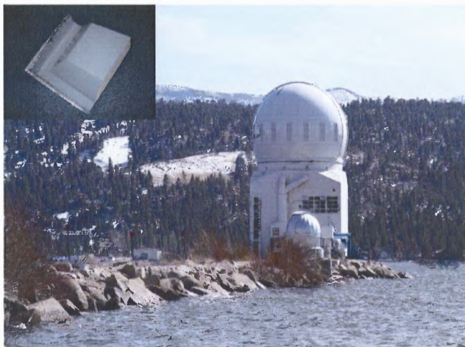
Figure 4.1 Image of new NST dome (MFG Ratech) dome with insert of foam core material
